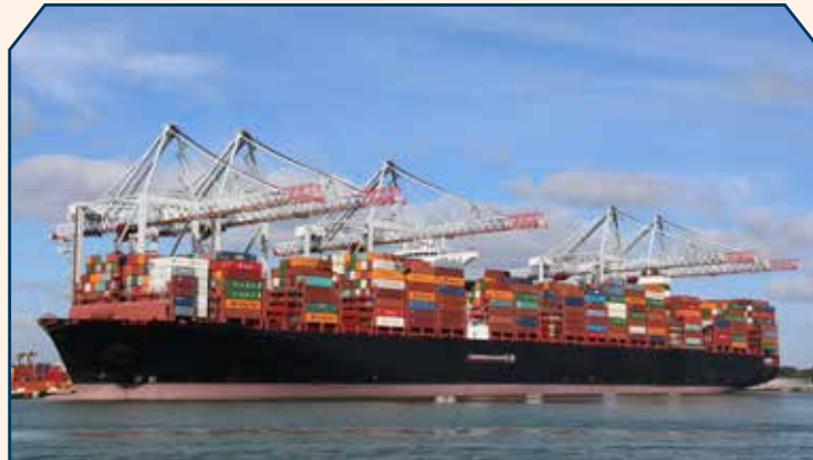
Awarding container cranes project in the commercial berth at Port of Duqm
