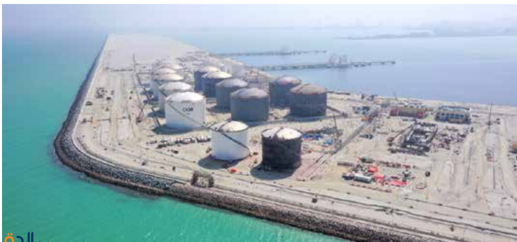
The oil berth at Duqm Port through which the project's products will be exported
