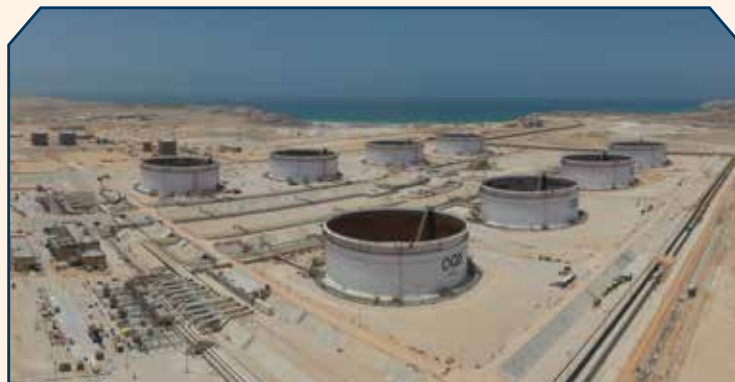
"OTTCO" puts final touches on the region's largest crude oil storage centre
